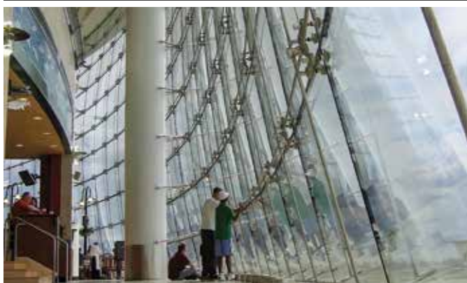
Example of a curved glass curtain wall at the Seattle-Tacoma International Airport.
