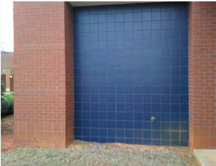
Figure 3: Exterior Wall at NBRC
