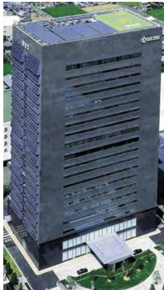
Kyocera headquarters building in Kyoto, Japan.
