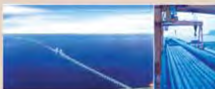
IMR develops various corrosion control methodologies and have been applying its techniques in industries. As an example, the Hangzhou Bay bridge with 36 km long used IMR's heavy corrosion protection coatings, cathodic protection tech., the corrosion sensors and in-situ monitoring techniques to insure 100 years lifetime.
