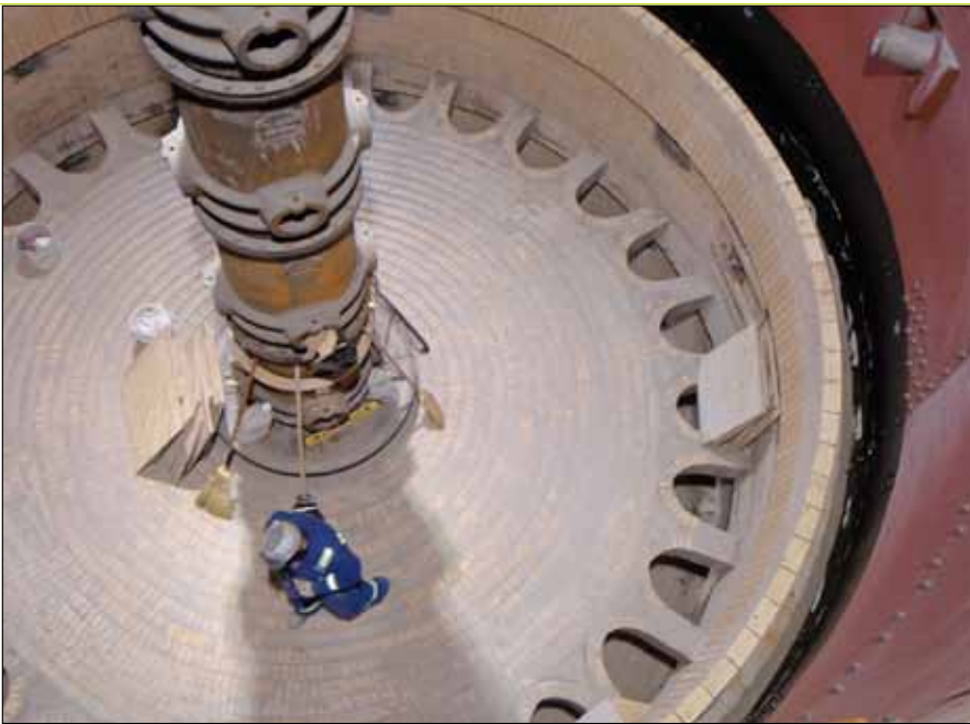
Refractory installation of a rotary hearth dome in western Canada.
