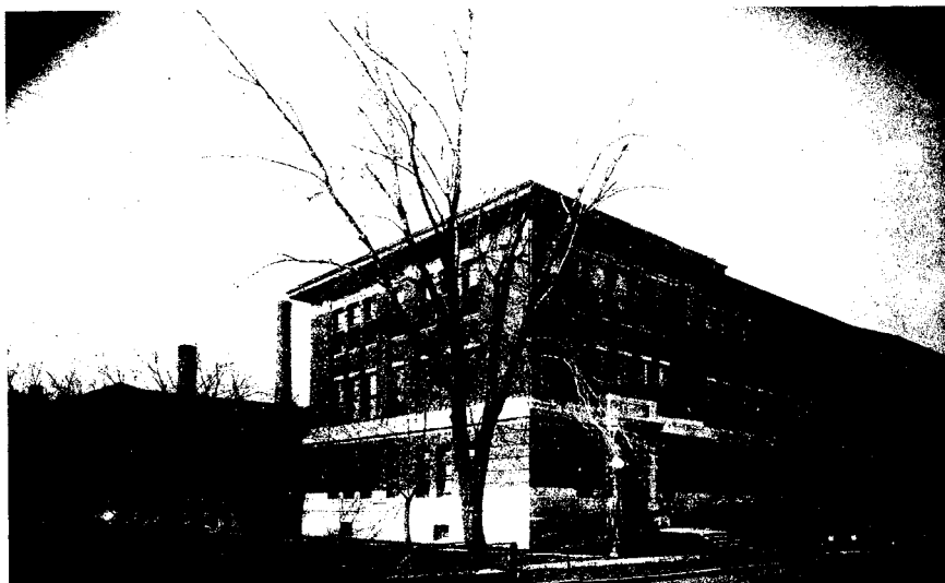
Ceramics Building (Built 1915-16) and Kiln in Rear (Built 1912). (Courtesy Am. Ceram. Soc.)
